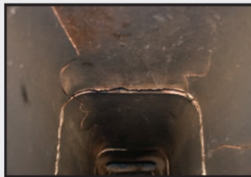
Actual photo of cracked flue tiles
