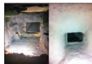
Before and after Chamber Coat
