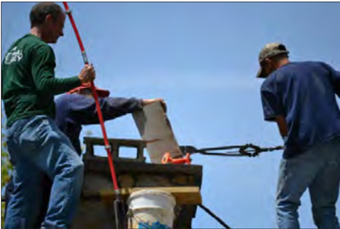
PterodacTILE removing concrete blocks.
