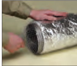
With one end of ArmorMesh clamped to the liner, pull the other end to snug along entire length.
