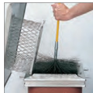
3. And clean the flue.
