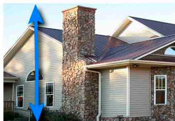
Photo 2 - Showing the House chimney (Ground to roof)
