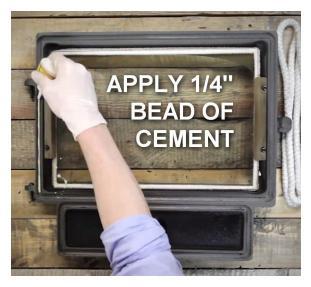
6. Apply a **1/4**" **bead** of gasket cement to the entire groove
