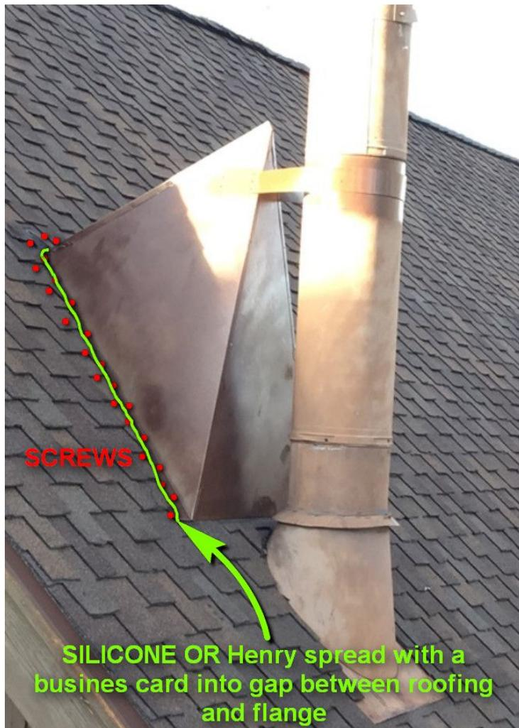
7. **Apply Silicone or Henry** into any gaps between the roofing material and the flange or ***splitter bottom!***
