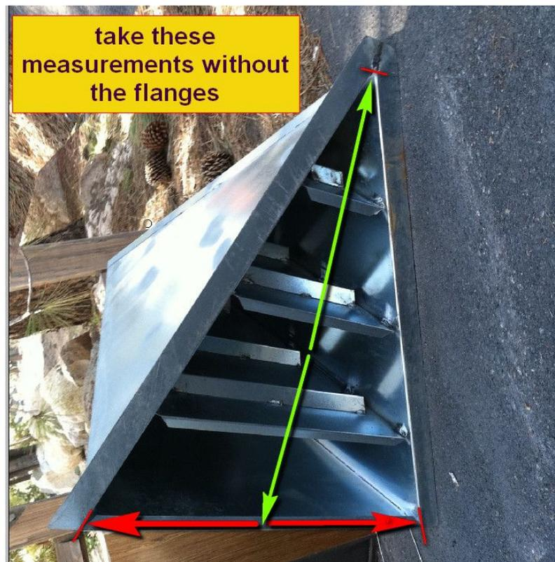
NOTE: We will want the splitter to end up as close to the chimney as possible. If the flashing is not installed yet - Remember that the flashing cone will take some room above where the chimney penetrates, so the bottom of the splitter will be right up against the flashing cone.
