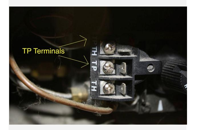
Then, unscrew the thermocouple from the valve (the copper colored tube):
