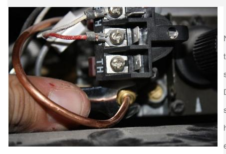
Next, you will have to test the magnet on the back side of the valve.
